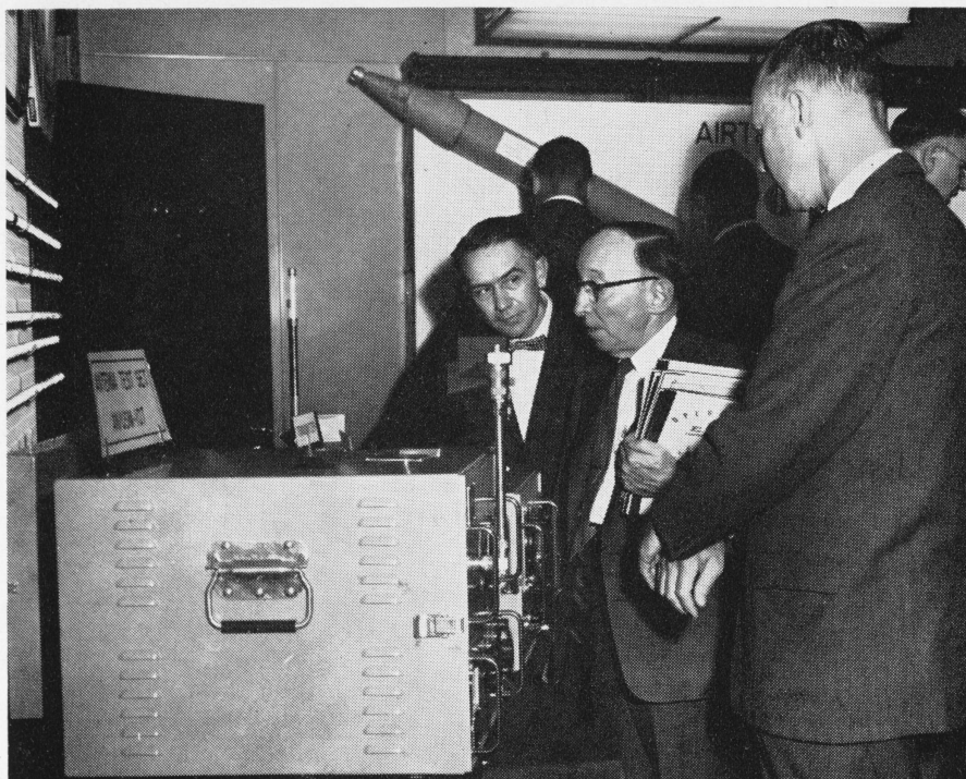
TUNING IN ON NEW PRODUCTS. President S. T. Williams and Airtronics engineers Frank Davis (left) and Lloyd Diehl (right) are examining an Antenna Test Set for calibrating and testing guided missile tracking antennas.
